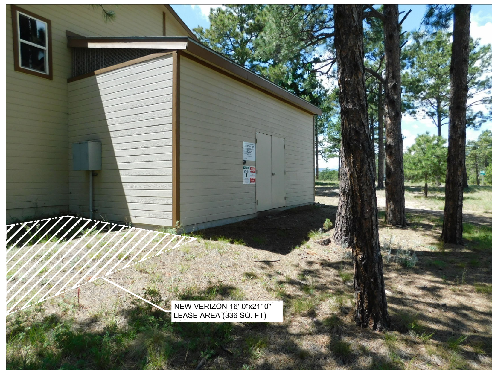
VIEW OF NEW LEASE AREA (LOOKING NORTHEAST)
