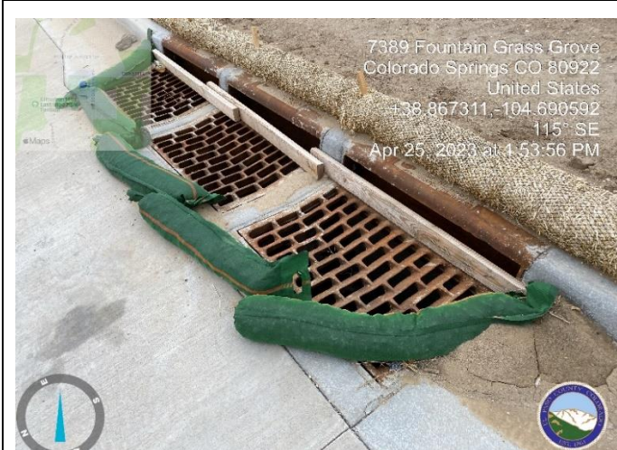
Photo 5: Maintenance Stormwater inlets as needed.
