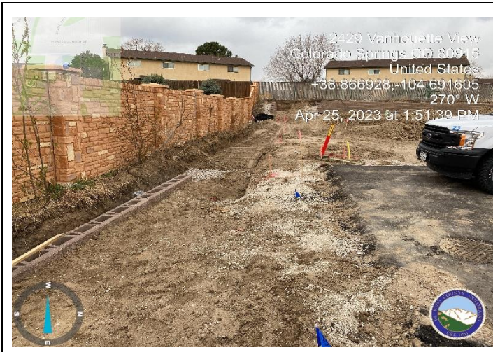
Photo 1: Swale A not completed. Missing retaining wall and concrete pan. (Page 3 of GEC)
