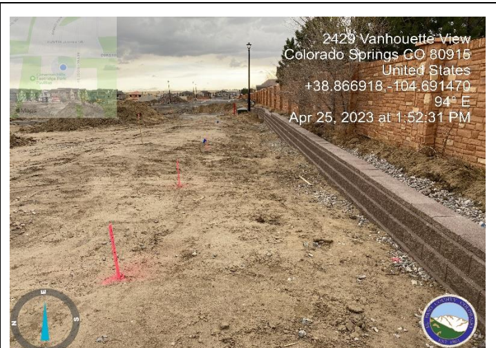
Photo 2: Swale A not completed. Missing retaining wall and concrete pan. (Page 3 of GEC) Concrete pan must extend and tie into rip rap run down.
