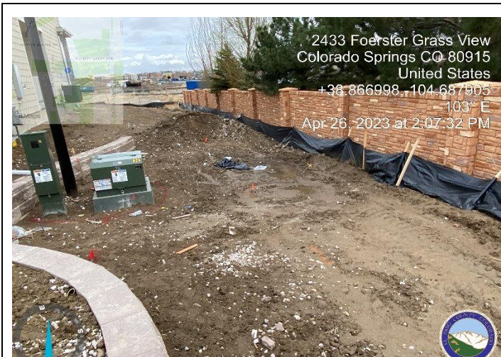
Photo 3: Swale C not completed per specification. (Swales are supposed to be 24' wide and clearance onsite is 17')
