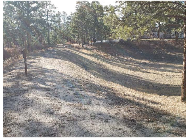
Detention Basin Along Deer Creek Road
