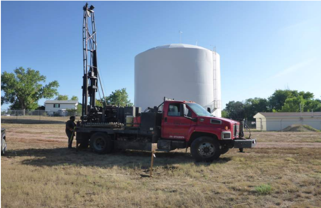
DRILLING BORING BP-3 - LOOKING SOUTH
