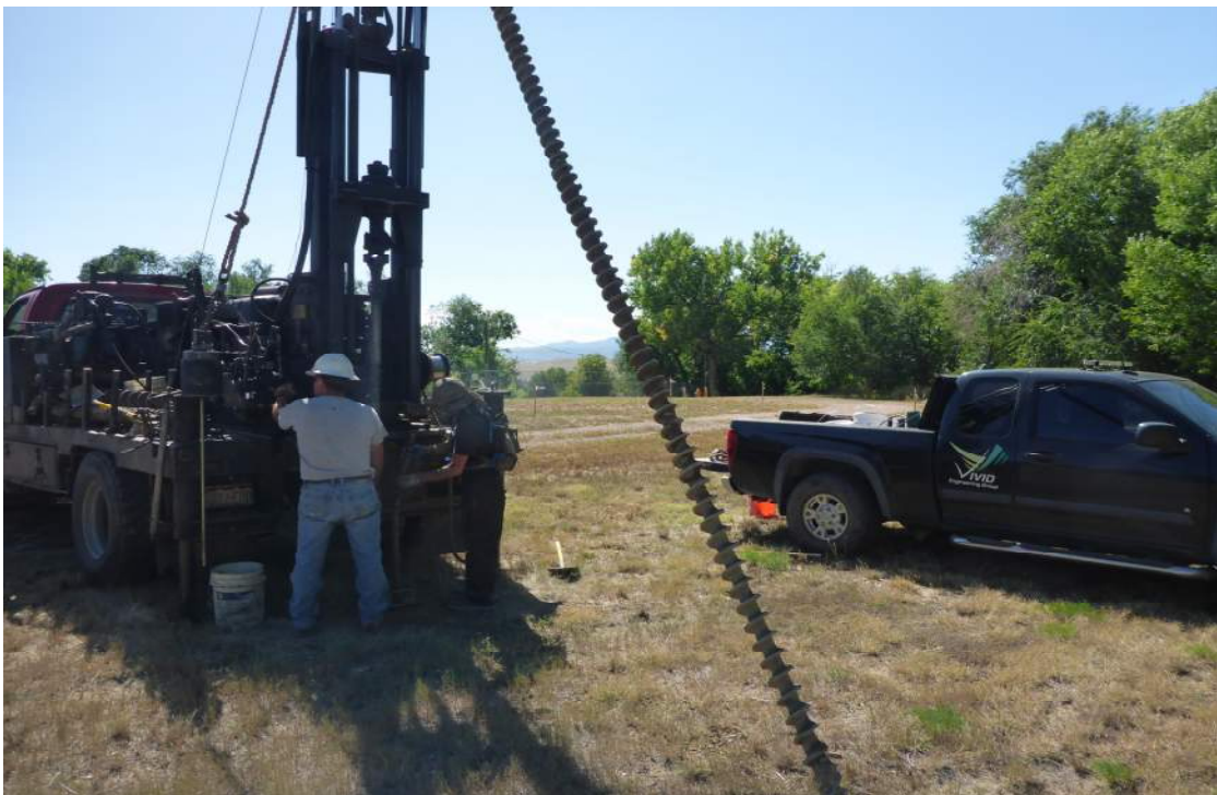
DRILLING BORING GEN-1 - LOOKING WEST
