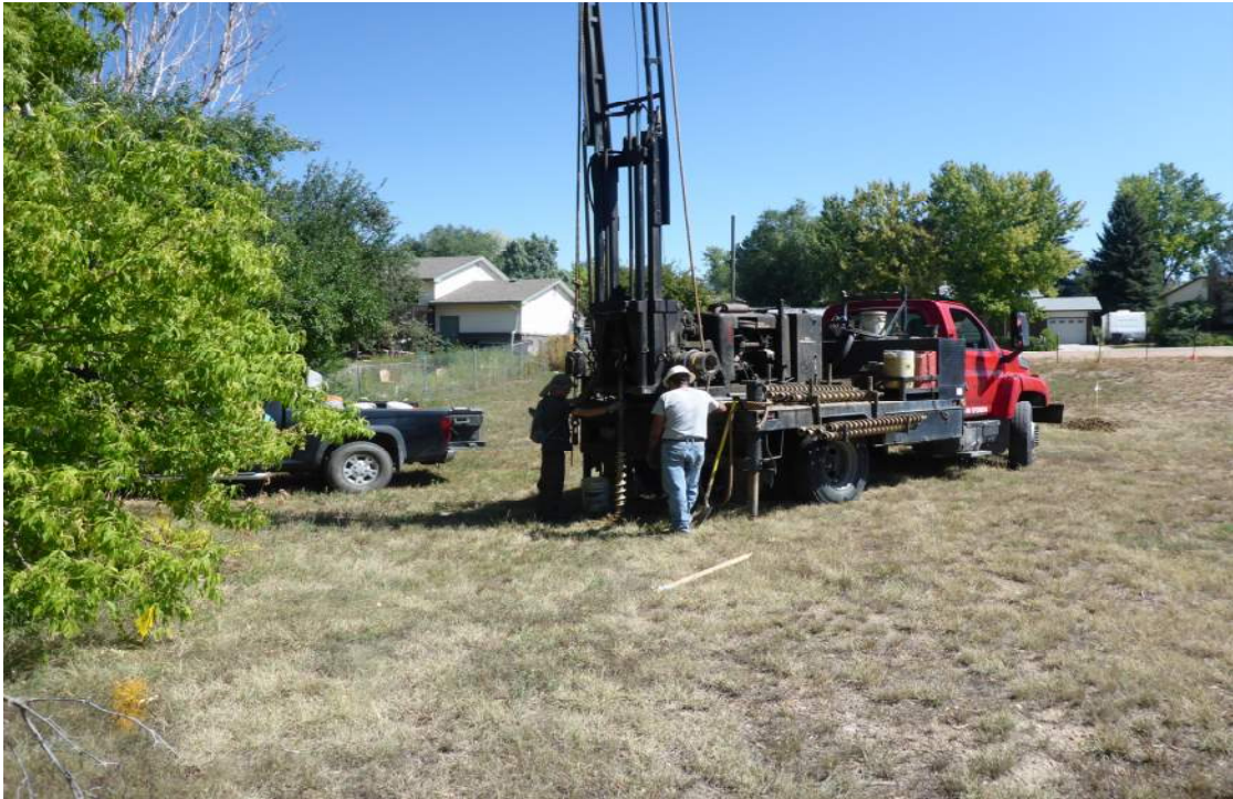
DRILLING BORING BP-1 - LOOKING EAST
