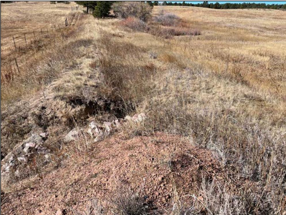
Photo 6 – Facing west from the southeast dam. Property line/fence is photo left, overflow channel is in the foreground, and detention area is photo right (no indicators of recent flow or flooding). A patch of sandbar willows behind the West swale dam is visible in the background. The Central swale edge is visible near the top right corner of the photo.
