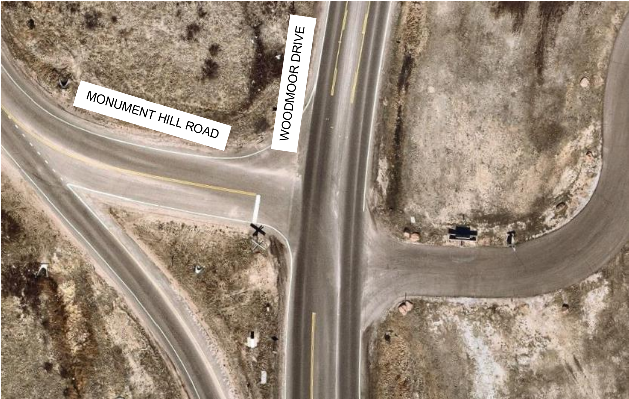
Monument Hill Road & Woodmoor Drive (#6)
