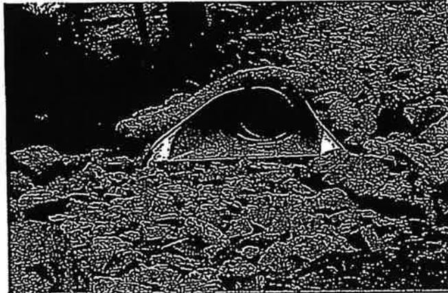
Photograph TOP-1. Riprap outlet protection.
