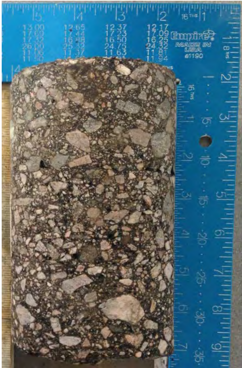
Pavement Core at SW-P-05 Eastbound lane, 7 inches thickness measured
