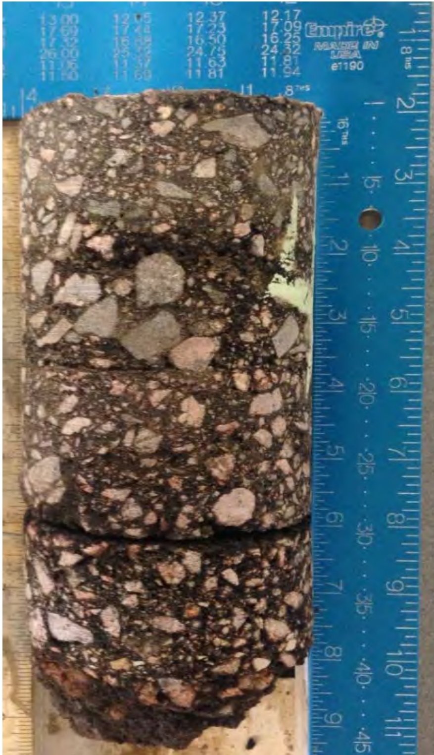
Pavement Core at SW-P-04 Westbound lane, 8 inches thickness measured
