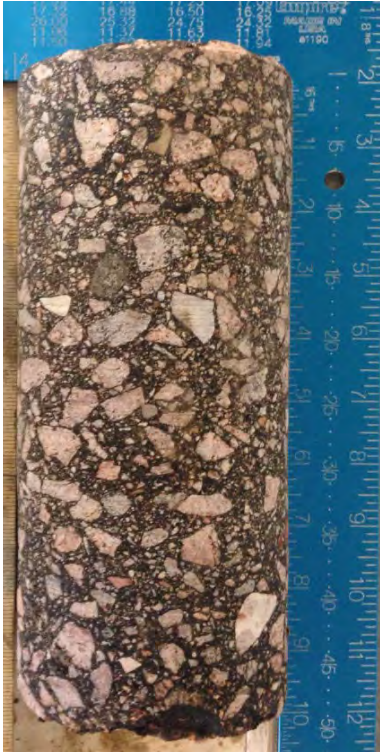
Pavement Core at SW-P-01 Eastbound lane, 9.5 inches thickness measured
