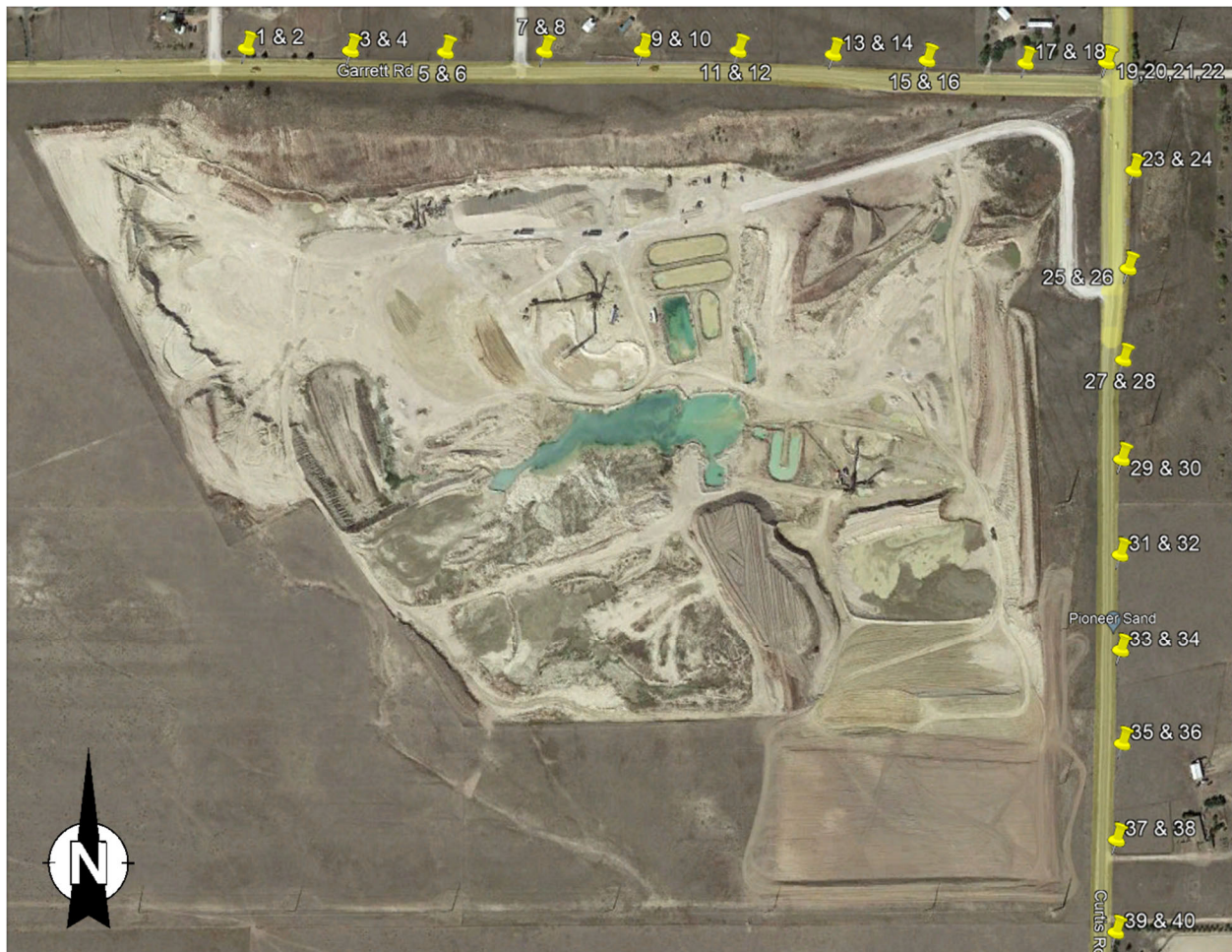
Figure 2: Road Condition Locations
