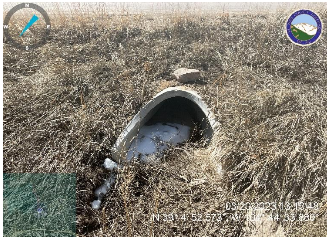
Photo 1: Remove vegetation from upgradient side of 18" culvert S1.
