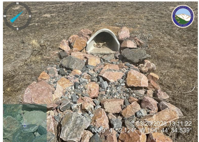
Photo 2: Remove sediment and fines from 23'L x10'W x 2' depth riprap apron of culvert S1.
