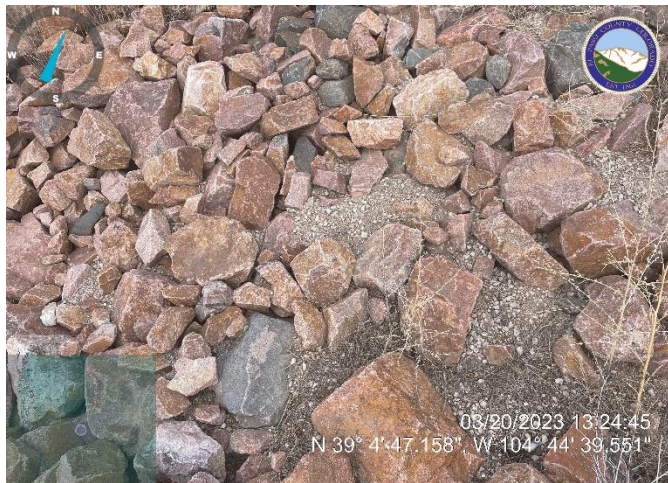
Photo 3: Remove sediment from riprap apron of culvert S2.
