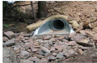
Photograph TOP-1. Riprap outlet protection.
