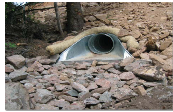
Photograph TOP-1. Riprap outlet protection.
