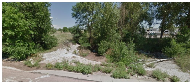
Figure 2: Curb Opening on North Half of the Galley Road Crossing (Looking to the North)
