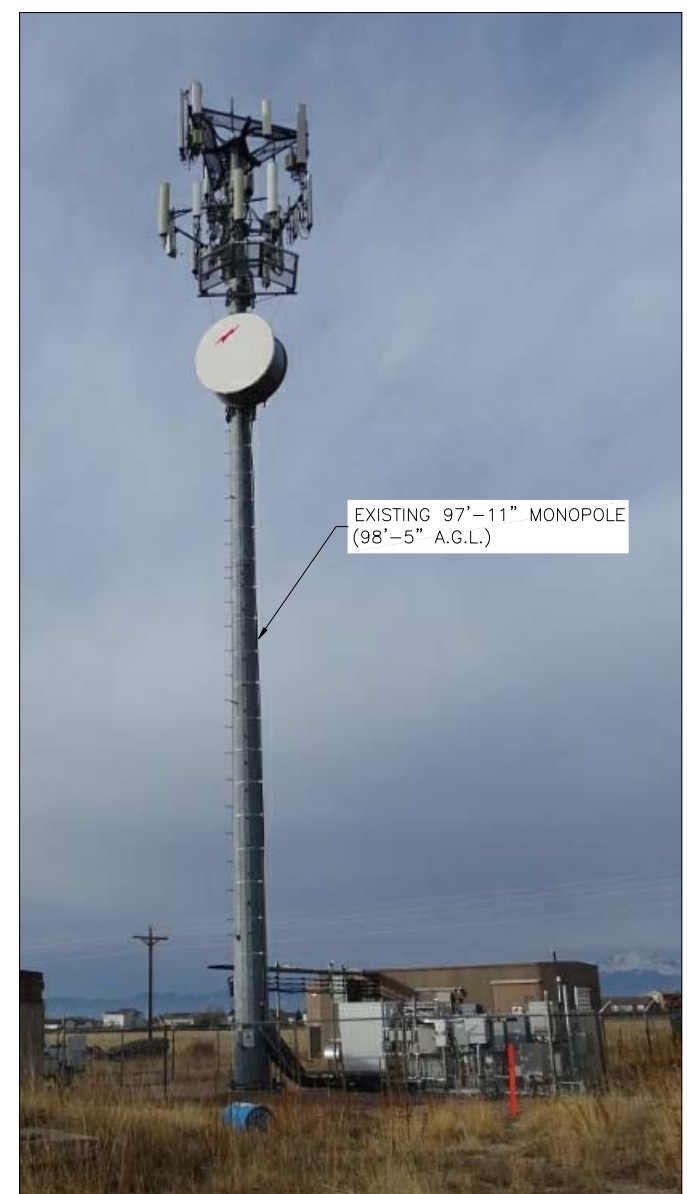
VIEW OF EXISTING MONOPOLE (LOOKING SOUTHWEST)
