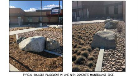
TYPICAL BOULDER PLACEMENT IN LINE WITH CONCRETE MAINTENANCE EDGE
