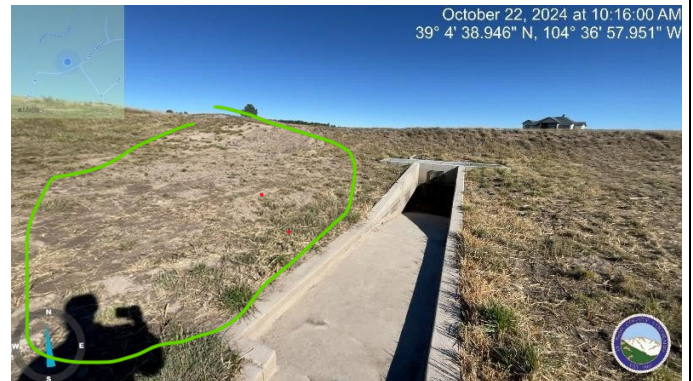
Photo 4: Detention pond D. Establish vegetation adjacent to outlet structure. Repair completed – see photo above.
