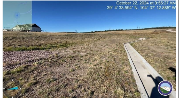
Photo 2: Detention Pond C. Establish vegetation in pond bottom. Repair completed – see photo above.
