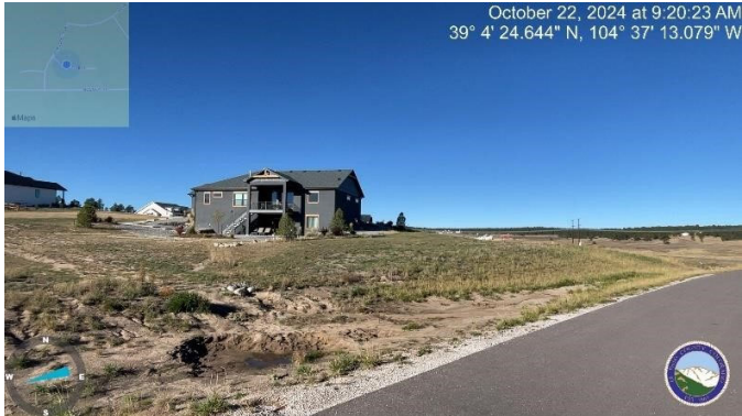
Photo 5: Sediment transfer at north side of lot 13 in drainage ditch needs to be removed and stabilized.
