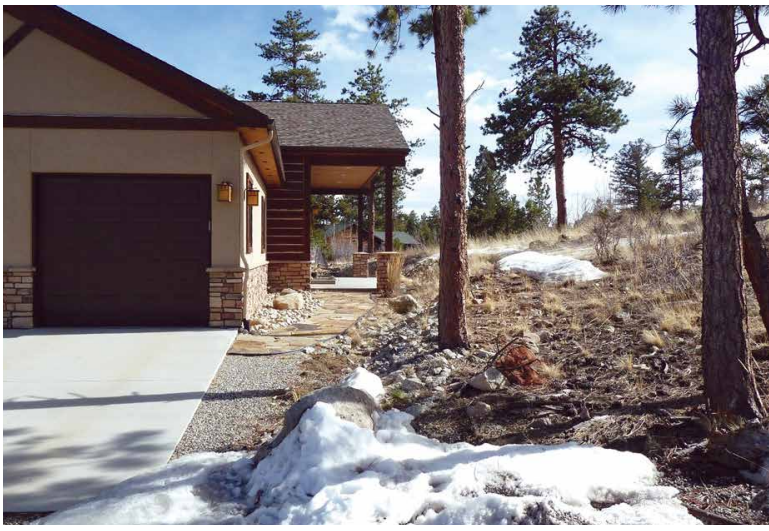
Top left: Hardening your home can include choosing noncombustible building materials like stucco paired with a stone facade. This house near Salida shows you don't have to sacrifice curb appeal to reduce the ignitability of your house. Photo: CSFS
