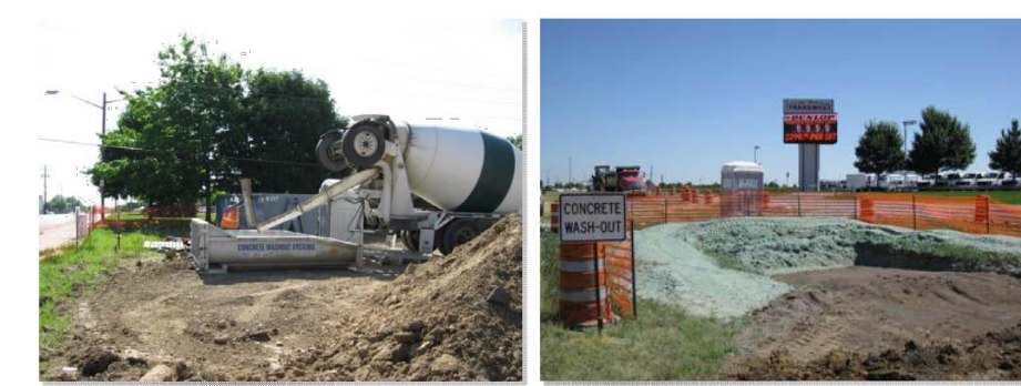
Photograph CWA-2. Prefabricated concrete washout. Photograph CWA-3. Earthen concrete washout.
