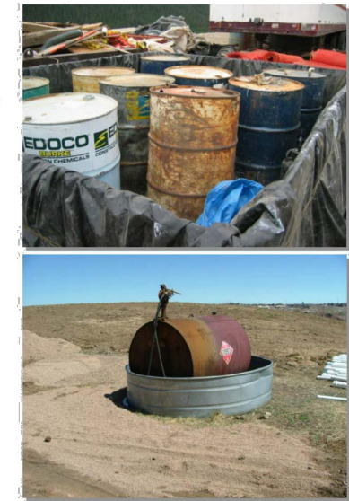
Photograph GH-1 and GH-2. Proper materials storage and secondary containment for fuel tanks are important good housekeeping practices.
