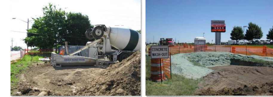
Photograph CWA-2. Prefabricated concrete washout. Photo courtesy of CDOT. Photograph CWA-3. Earthen concrete washout. Photo courtesy of CDOT.
