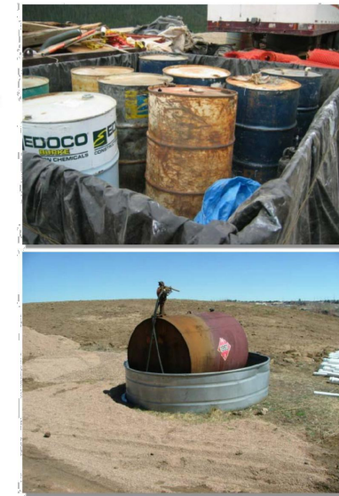
Photograph GH-1 and GH-2. Proper materials storage and secondary containment for fuel tanks are important good housekeeping practices. Photos courtesy of CDDP and City of Aurora.
