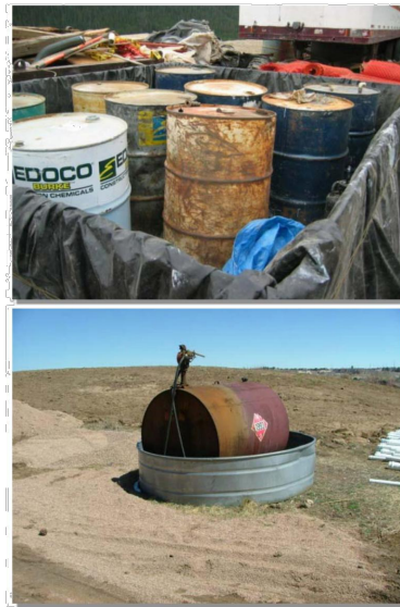
Photographs GH-1 and GH-2. Proper material staging and secondary containment for fuel tanks are important good housekeeping practices. Photos courtesy of CDOT and City of Aurora.
