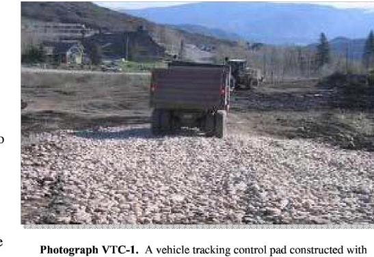
Photograph VTC-1. A vehicle tracking control pad constructed with properly sized rock reduces off-site sediment tracking.
