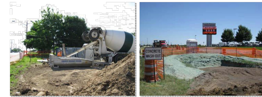
Photograph CWA-2. Prefabricated concrete washout. Photo courtesy of CDOT.
