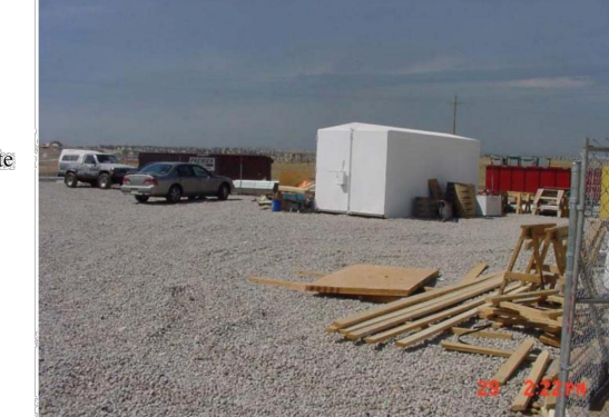
Photograph SSA-1. Example of a staging area with a gravel surface to prevent mud tracking and reduce runoff. Photo courtesy of Douglas County.
