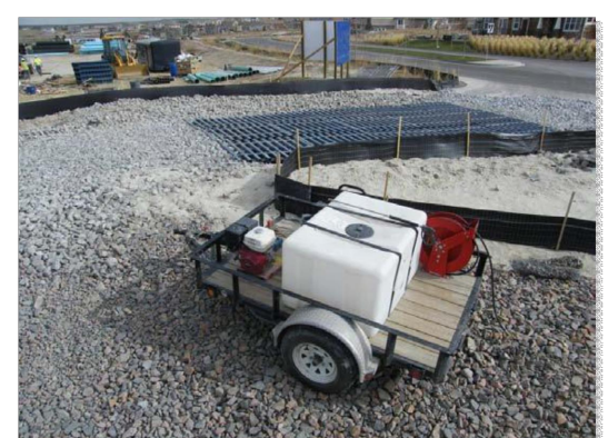
Photograph VTC-2. A vehicle tracking control pad with wheel wash facility. Photo courtesy of Tom Gies.
