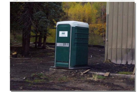
Photograph GH-3. Locate portable toilet facilities on level surfaces away from waterways and storm drains. Photo courtesy of WVI.
