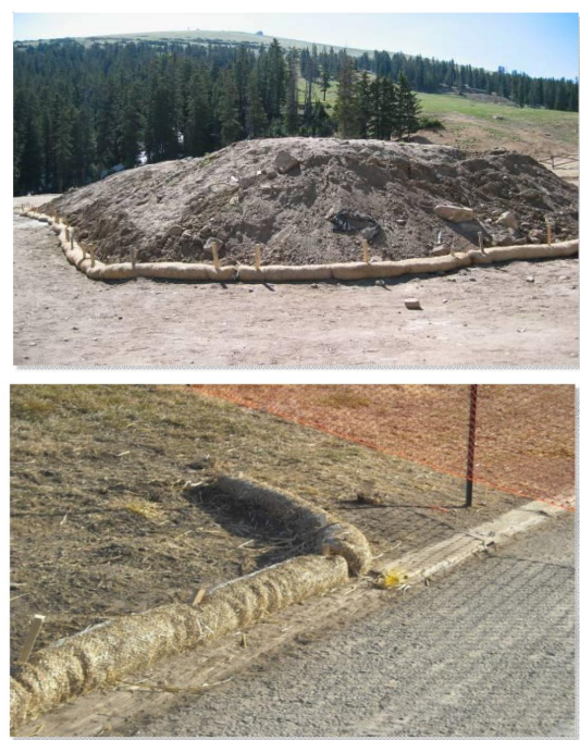
Photographs SCL-1 and SCL-2. Sediment control logs used as 1) a perimeter control around a stockpile and, 2) as a "J-hook" perimeter control at the corner of a construction site.
