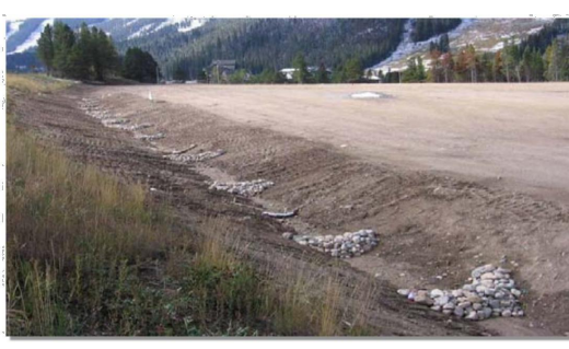
Photograph CD-1. Rock check dams in a roadside ditch. Photo courtesy of WVE.
