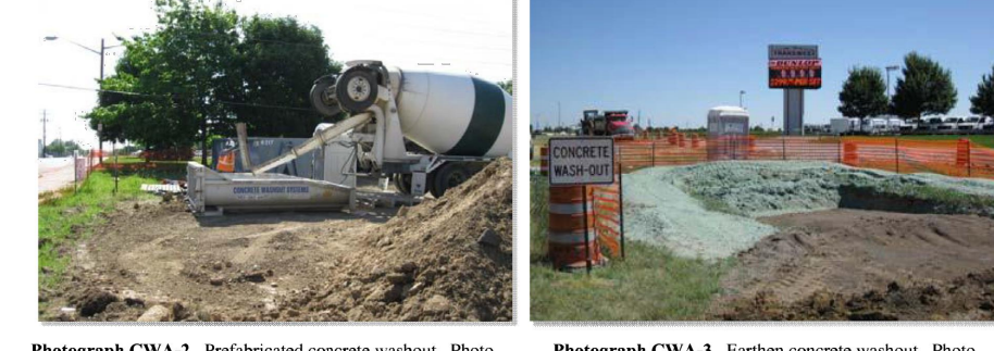
Photograph CWA-2. Prefabricated concrete washout. Photograph CWA-3. Earthen concrete washout.
