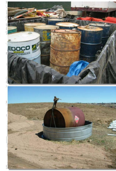
Photographs GH-1 and GH-2. Proper materials storage and secondary containment for fuel tanks are important good housekeeping practices. Photos courtesy of CDDP and City of Aurora.
