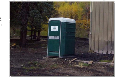
Photograph GH-3. Locate portable toilet facilities on level surfaces away from waterways and storm drains. Photo courtesy of WVE.
