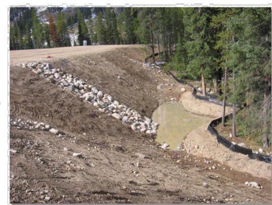
Photograph SB-1. Sediment basin at the toe of a slope. Photo courtesy of WWH.
