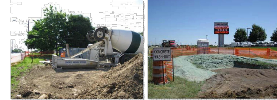
Photograph CWA-2. Prefabricated concrete washout. Photo courtesy of CDOT. Photograph CWA-3. Earthen concrete washout. Photo courtesy of CDOT.
