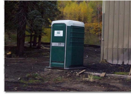
Photograph GH-3. Locate portable toilet facilities on level surfaces away from waterways and storm drains. Photo courtesy of WVE.
