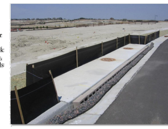
Photograph IP-4. Inlet protection for a curb opening inlet.
