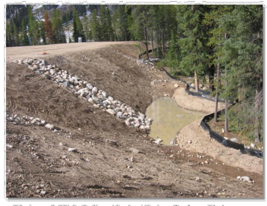
Photograph SB-1. Sediment basin at the toe of a slope. Photo courtesy of WWTB.
