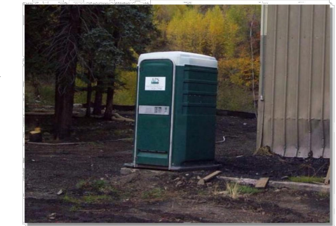
Photograph GH-3. Locate portable toilet facilities on level surfaces away from waterways and storm drains.
