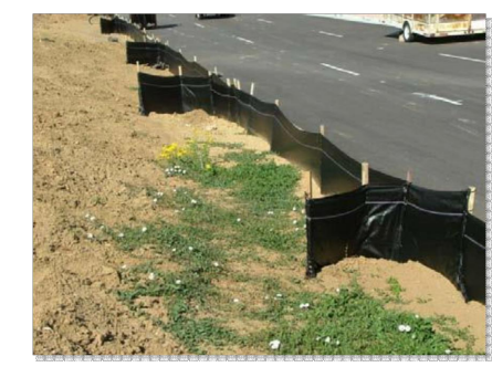
Photograph SF-2. When silt fence is not installed along the contour, a 'J-hook' installation may be appropriate to ensure that the BMP does not create concentrated flow parallel to the silt fence. Photo courtesy of Tom Ore.
