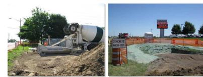
Photograph CWA-2. Prefabricated concrete washout. Photo courtesy of CDOT.
