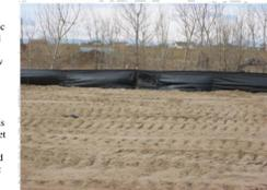
**Photograph SF-1.** Silt fence creates a sediment barrier, forcing sheet flow runoff to evaporate or infiltrate.
