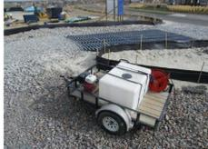
Photograph VTC-2. A vehicle tracking control pad with wheel wash facility. Photo courtesy of Tom Gore.
