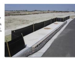
Inlet protection consists of permeable barriers installed around an inlet to filter runoff and remove sediment prior to entering a storm drain inlet. Inlet protection can be constructed from rock socks, sediment control logs, silt fence, block and rock socks, or other materials approved by the local jurisdiction. Area inlets can also be protected by over-excavating around the inlet to form a sediment trap.
