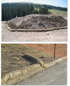
**Photographs SCL-1 and SCL-2.** Sediment control logs used as 1) a perimeter control around a stockpile and, 2) as a "J-hook" perimeter control at the corner of a construction site.
