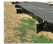
**Photograph SF-2.** When silt fence is not installed along the contour, a "J-hook" installation may be appropriate to ensure that the BMP does not create concentrated flow parallel to the silt fence. Photo courtesy of Tom Gore.
