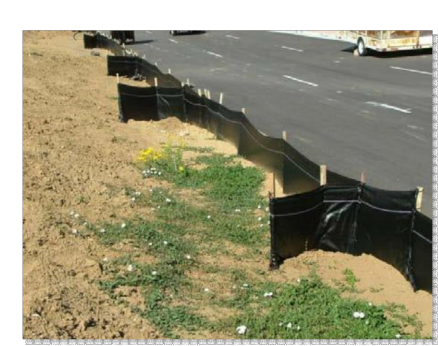
Photograph SF-2. When silt fence is not installed along the contour, a "J-hook" installation may be appropriate to ensure that the BMP does not create concentrated flow parallel to the silt fence. Photo courtesy of Tom Owe.
