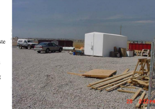
Photograph SSA-1. Example of a staging area with a gravel surface to prevent mud tracking and reduce runoff. Photo courtesy of Douglas County.
