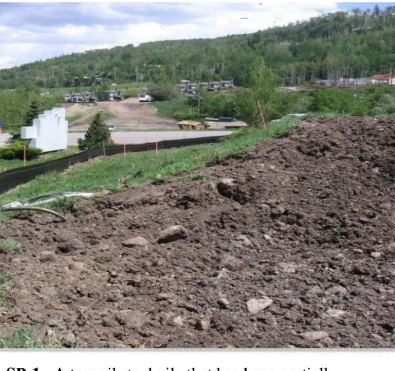
Photograph SP-1. A topsoil stockpile that has been partially revegetated and is protected by silt fence perimeter control.
