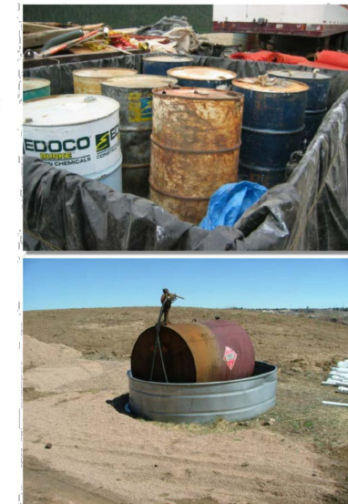
Photographs GH-1 and GH-2. Proper materials storage and secondary containment for fuel tanks are important good housekeeping practices. Photos courtesy of CDDP and City of Aurora.
