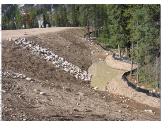
Photograph SB-1. Sediment basin at the top of a slope. Photo courtesy of UFWI.
