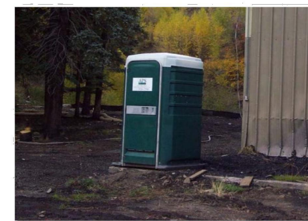
Photograph GH-3. Locate portable toilet facilities on level surfaces away from waterways and storm drains. Photo courtesy of WVI.
