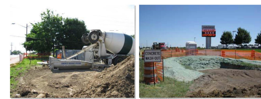
Photograph CWA-2. Prefabricated concrete washout. Photo courtesy of CDOT. Photograph CWA-3. Earthen concrete washout. Photo courtesy of CDOT.
