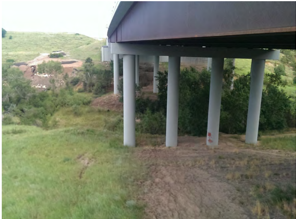
POWERS BLVD BRIDGE LOOKING NORTH
