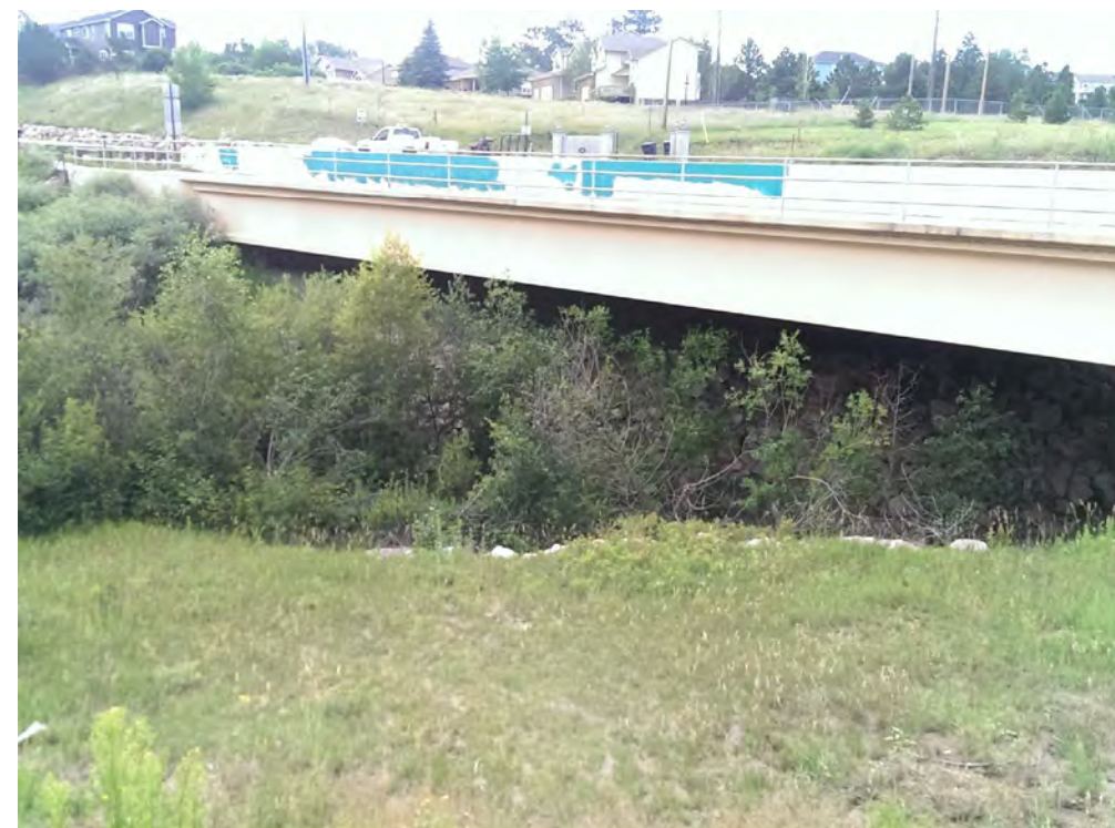
OLD RANCH ROAD BRIDGE LOOKING NORTH
