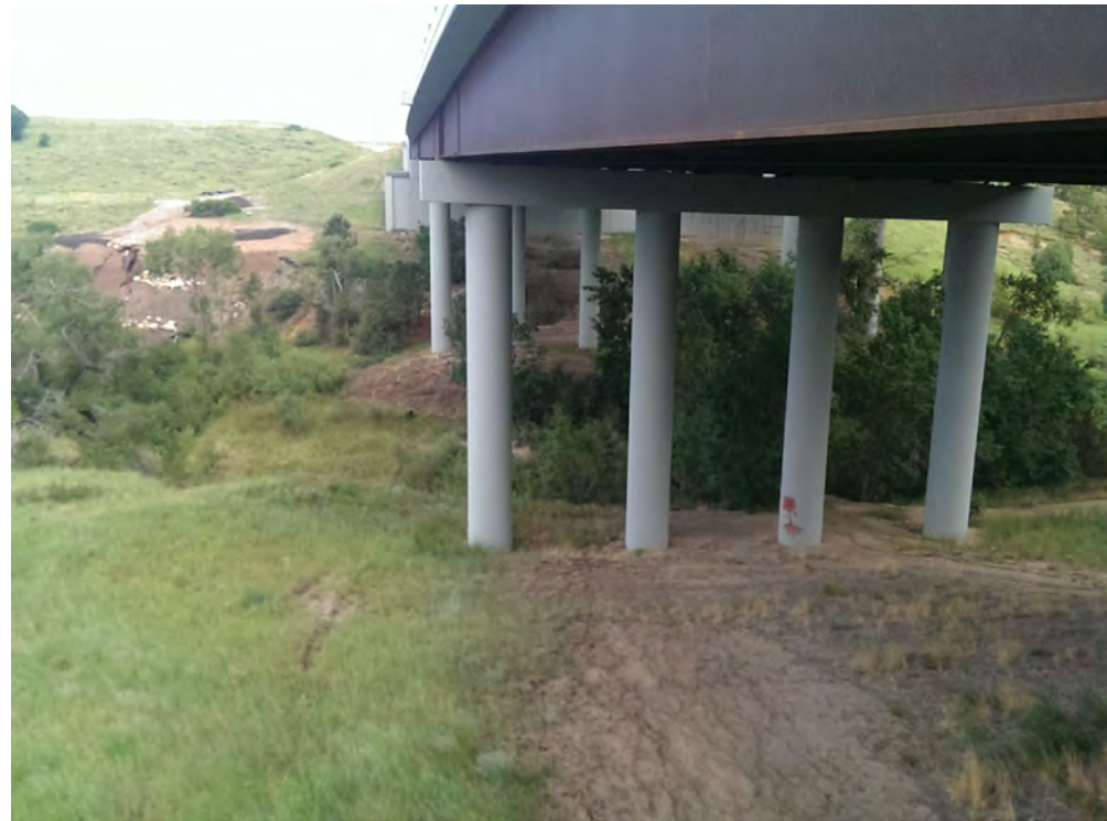
POWERS BLVD BRIDGE LOOKING NORTH
