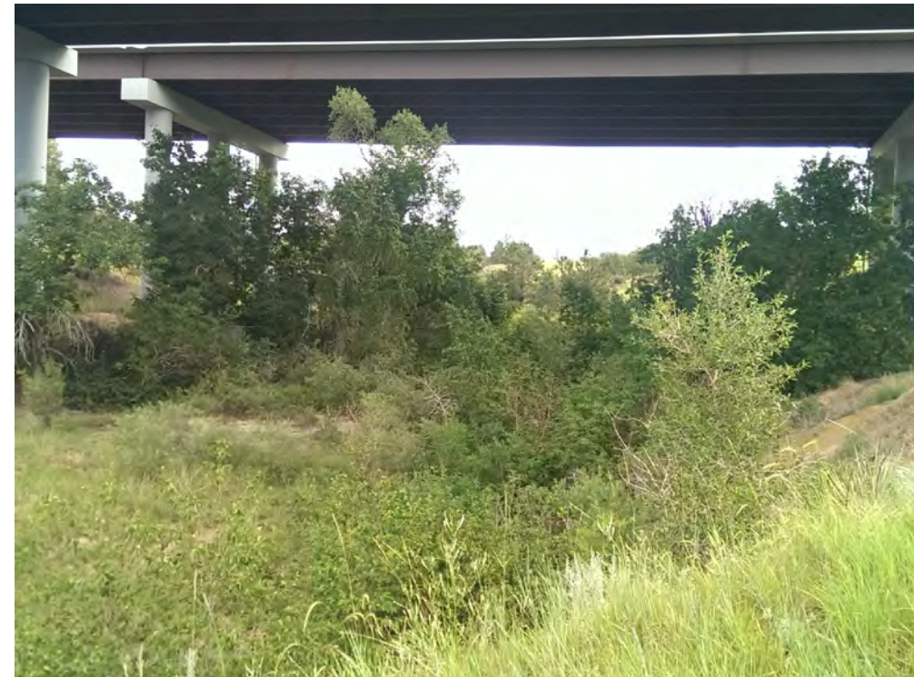
POWERS BLVD BRIDGE LOOKING UPSTREAM
