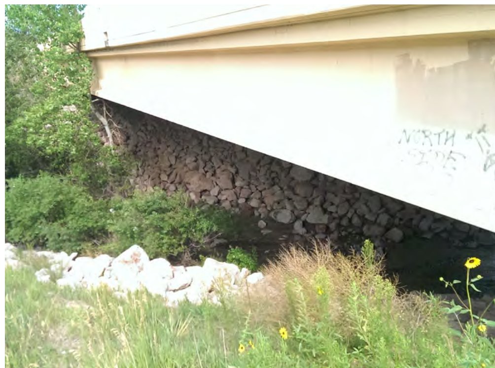
OLD RANCH ROAD BRIDGE DOWNSTREAM
