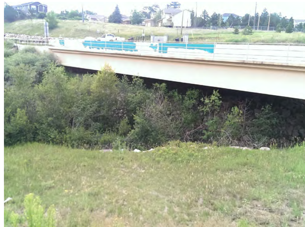
OLD RANCH ROAD BRIDGE LOOKING NORTH
