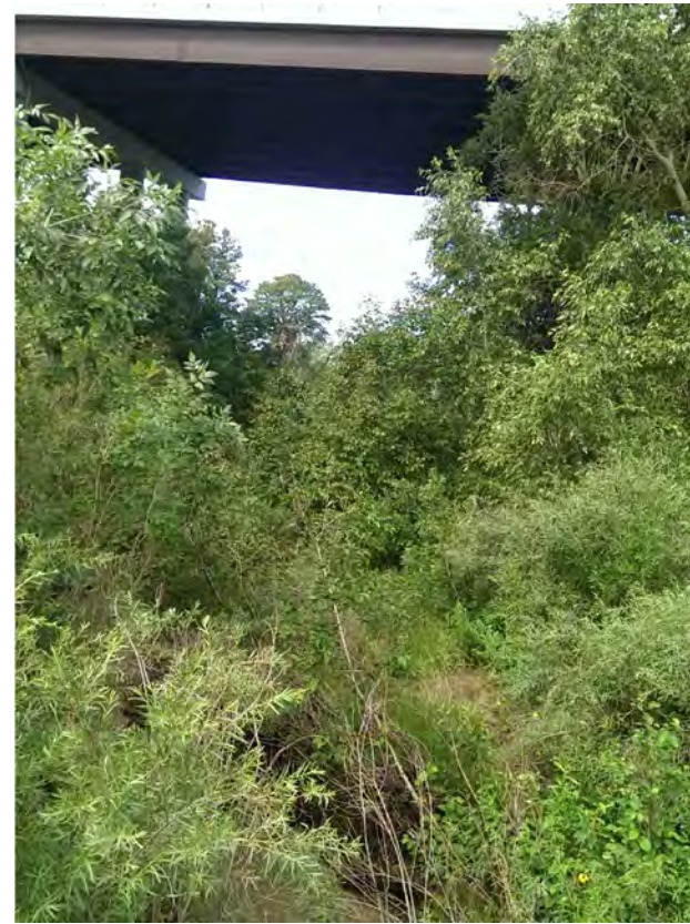
CHANNEL CONDITIONS APPROX. STA 165+00
