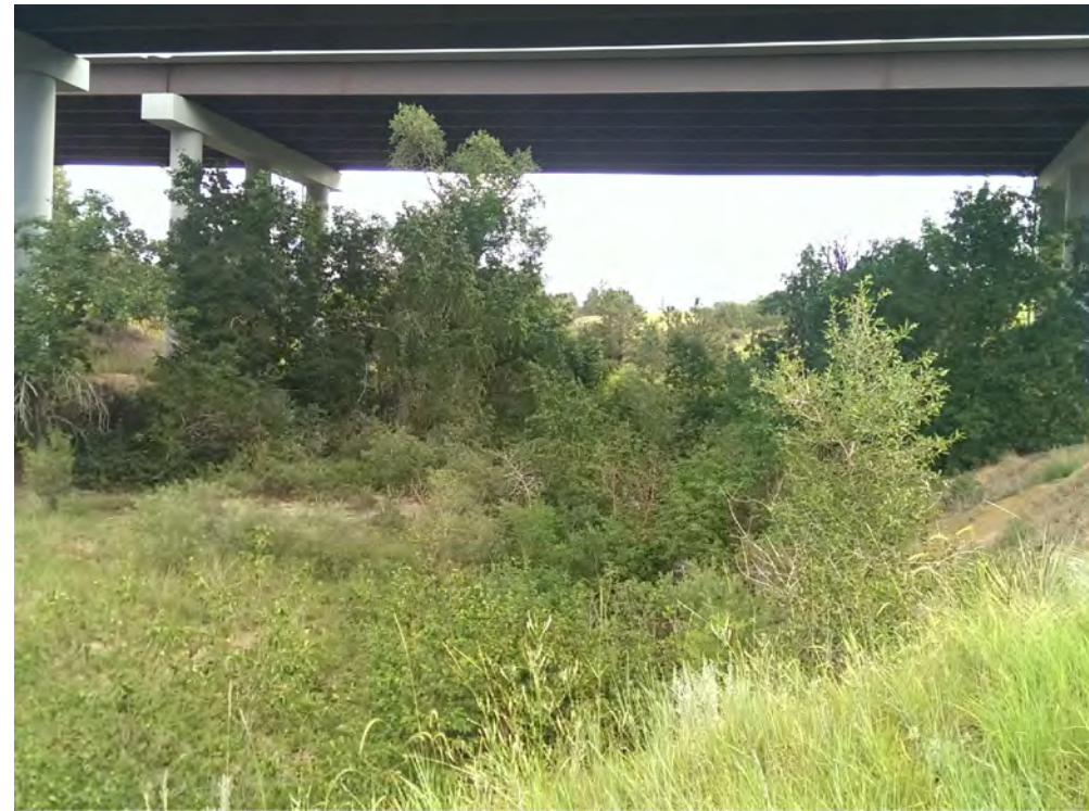
POWERS BLVD BRIDGE LOOKING UPSTREAM
