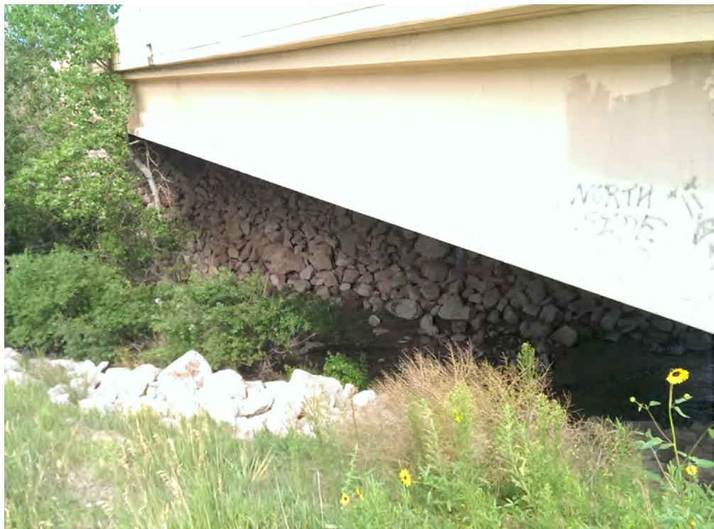
OLD RANCH ROAD BRIDGE DOWNSTREAM
