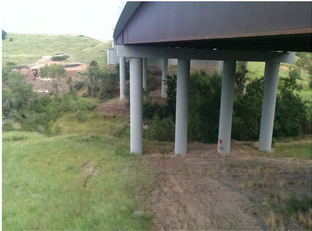
POWERS BLVD BRIDGE LOOKING NORTH
