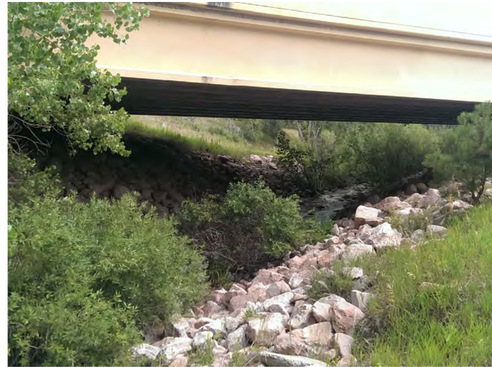
OLD RANCH ROAD BRIDGE LOOKING UPSTREAM
