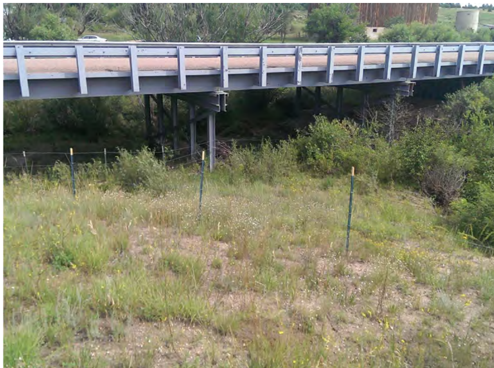
OTERO AVE BRIDGE LOOKING UPSTREAM
