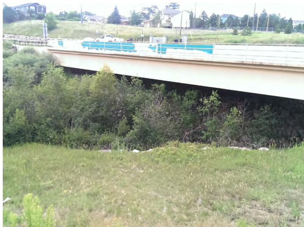
OLD RANCH ROAD BRIDGE LOOKING NORTH
