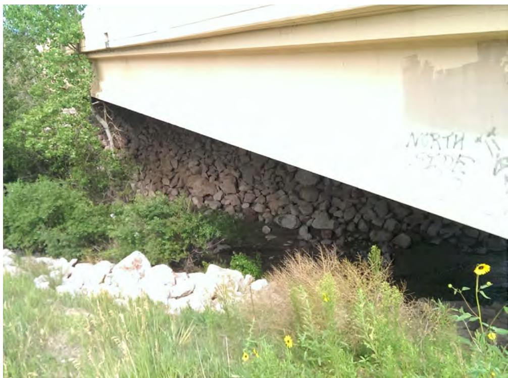
OLD RANCH ROAD BRIDGE DOWNSTREAM
