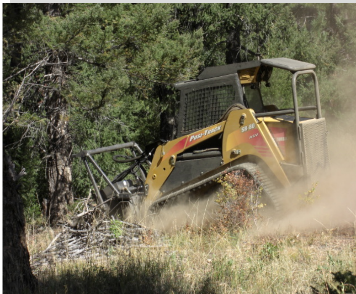
Machine mastication with skid steer
