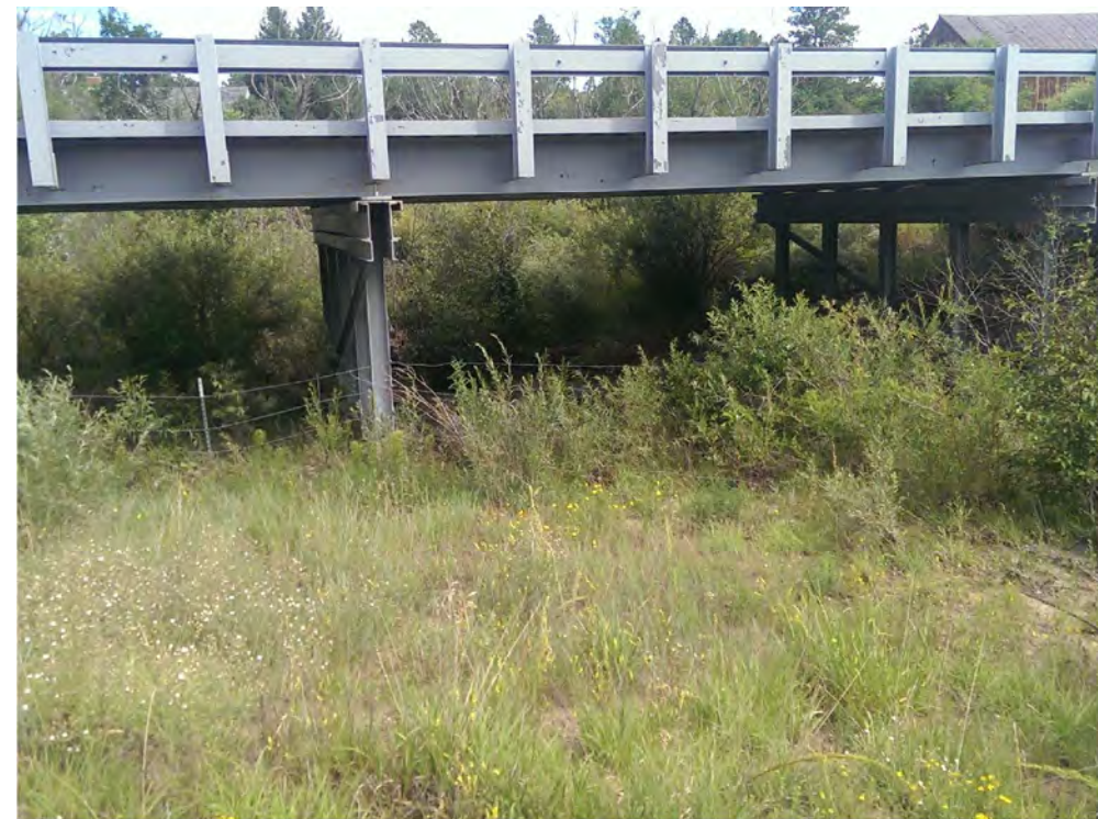
OTERO AVE BRIDGE LOOKING UPSTREAM
