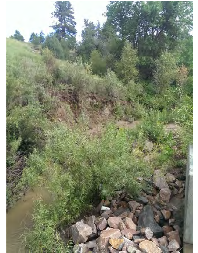
CHANNEL CONDITIONS APPROX. STA 175+00
