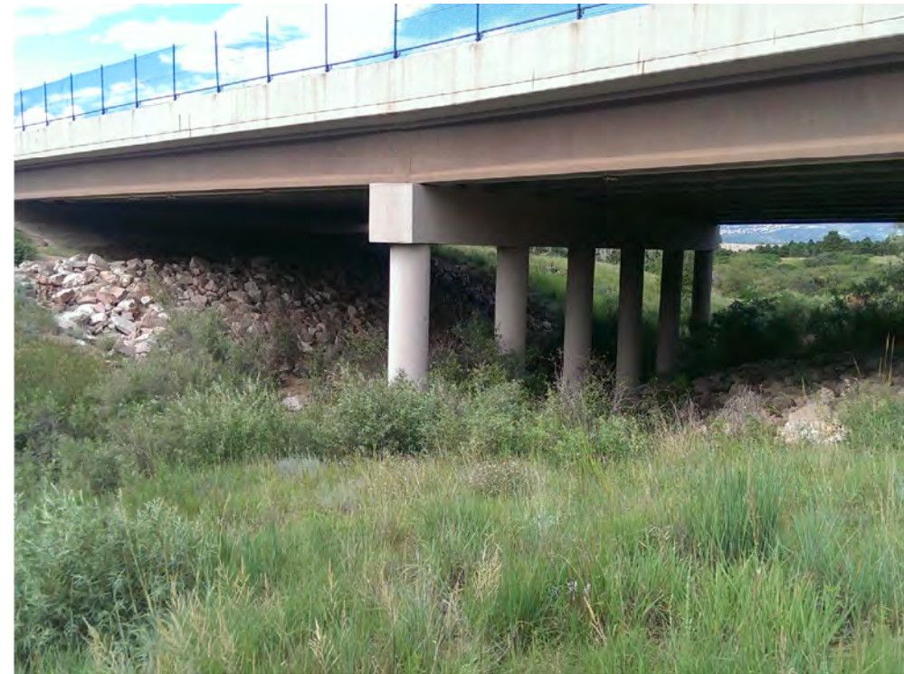
HWY 83 BRIDGE LOOKING UPSTREAM
