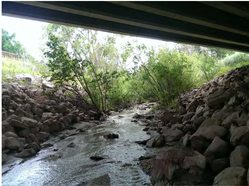
OLD RANCH ROAD BRIDGE LOOKING UPSTREAM
