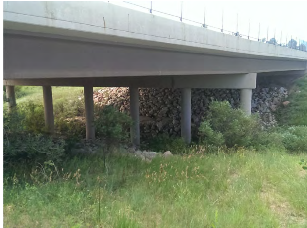
HWY 83 BRIDGE LOOKING NORTH
