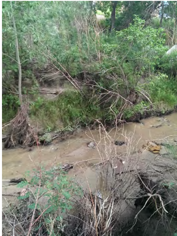
CHANNEL CONDITIONS APPROX. STA 169+00
