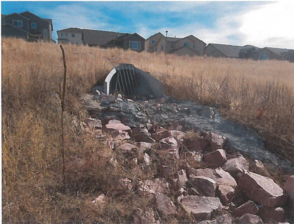
48" stormwater outlet in the eastern side of the site.
