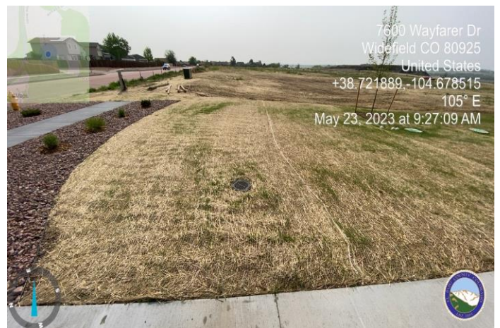
Photo 4: Grade to promote positive drainage to area drain
