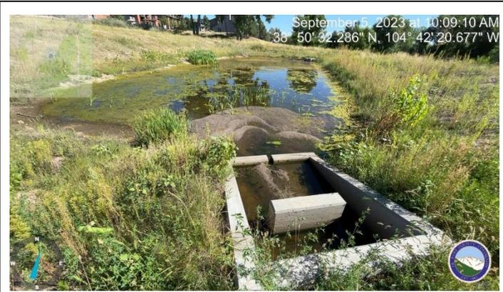
Photo 3: Detention Pond forebay. Sediment needs to be cleaned out and disposed of.
