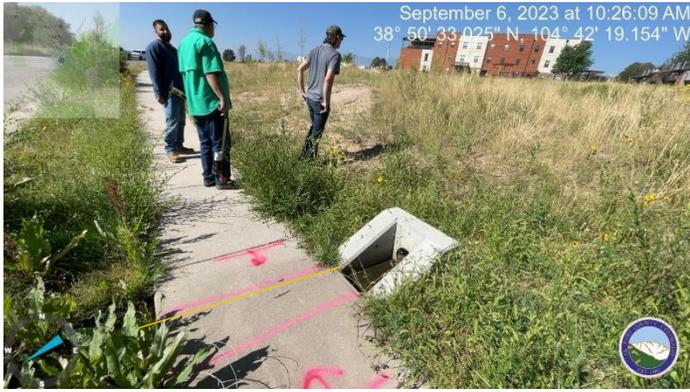
Photo 5: Concrete chase is not installed per plan.
