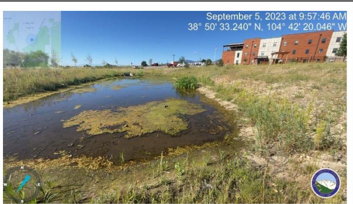
Photo 2: Detention Pond is holding water. Sediment from embankment has filled in floor of pond. Clean out and dispose of sediment throughout.
