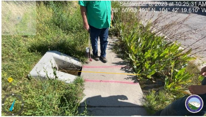
Photo 6: Concrete chase is not installed per plan.
