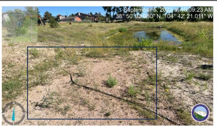
Photo 4: Maintenance access road. Per plan needs to be 11' wide and 1' thickness. Reestablish.
