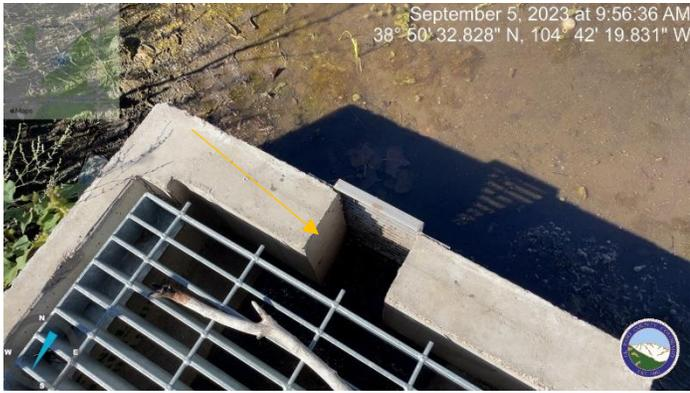
Photo 7: Outlet structure is missing the orifice plate and neoprene gasket per approved plans.
