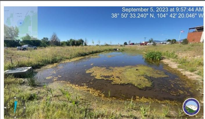
Photo 1: Detention Pond is holding water. Discrepancy in elevation at outfall structure. Reference notes above.
