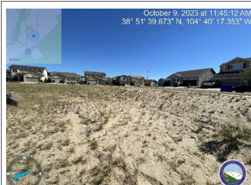
Photo 5: Sparse vegetation on the east banks of Trickle channel is causing erosion. Sediment from slopes needs to be cleaned out of channel.
