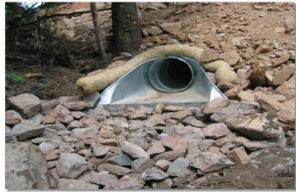
Photograph TOP-1. Riprap outlet protection.
