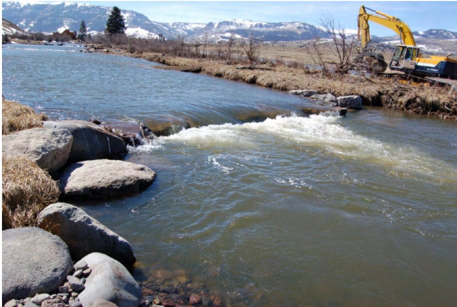
Figure A.14. Cross vane.
