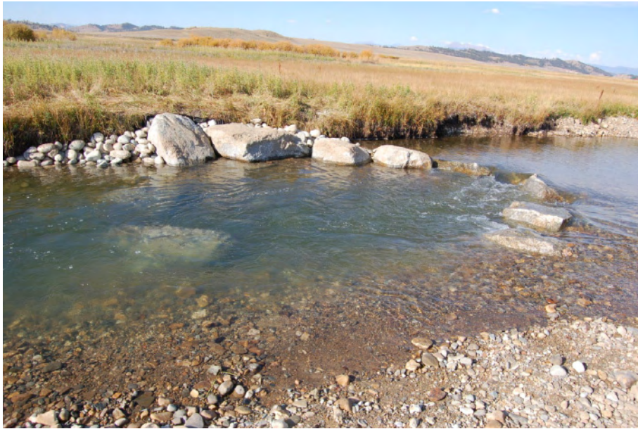
Figure A.6. Excavate a pool.
