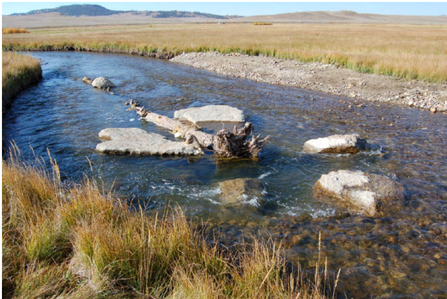
Figure A.23. Mid-channel root wad/log.
