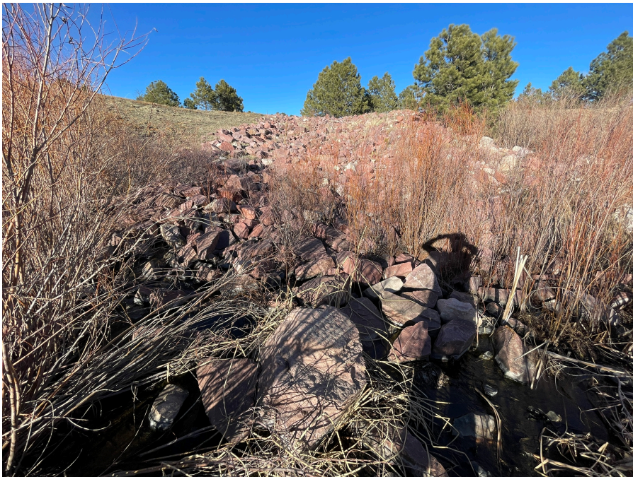
Pond 2 Emergency Spillway Looking upstream (northeast)
