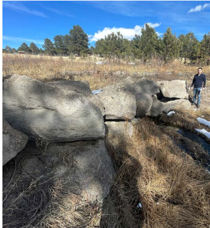
0030 E Boulder dam in place & stable for 40+ years
