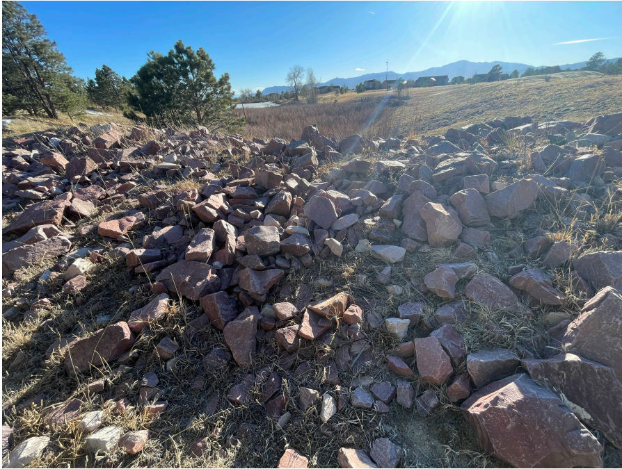
Pond 2 Emergency Spillway Looking downstream (southwest)
