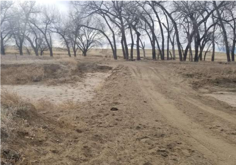
33. Drainage located on the east end of property looking west.
