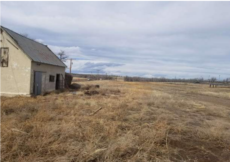
3. Southwest corner of property looking northwest with stable structure/barn. Stucco exterior.
