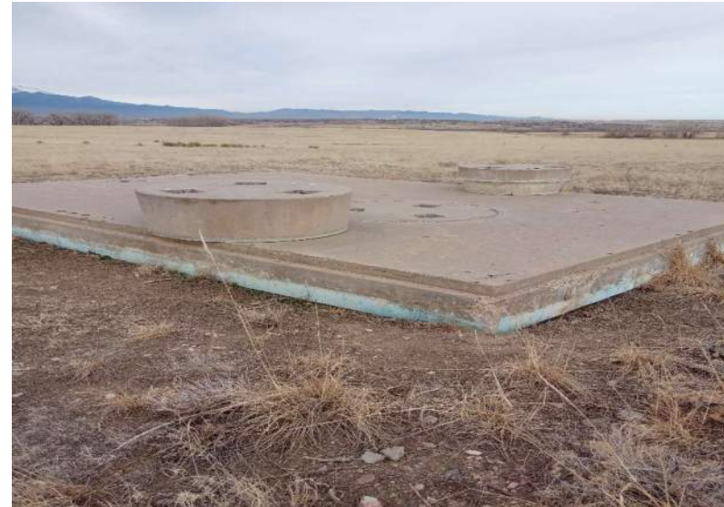
17. Foundation identified at the Site of an unknown utility structure.
