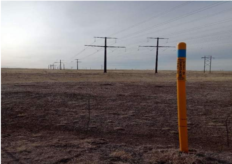
16. Petroleum line crossing north portion of the Site near Bradley Road.
