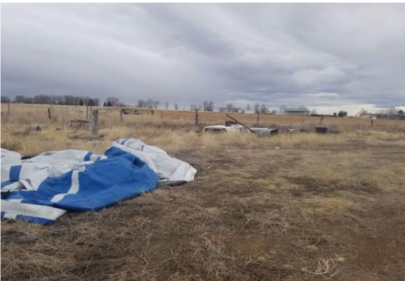
50 Debris on southwest center property boundary.
