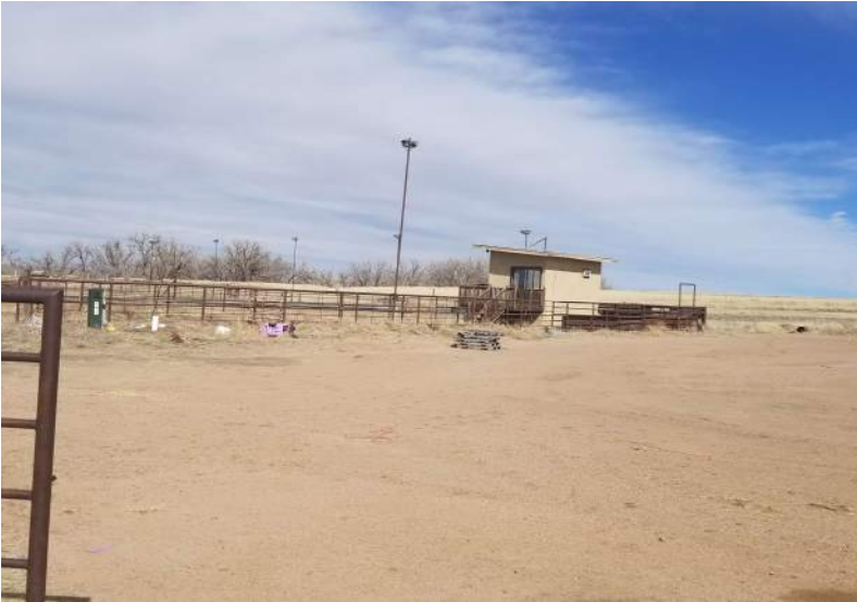
9. Equestrian center and existing announcer's building.
