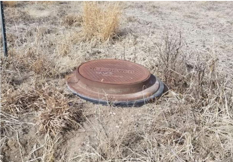
15. Storm sewer or sanitary sewer on west end of Site.
