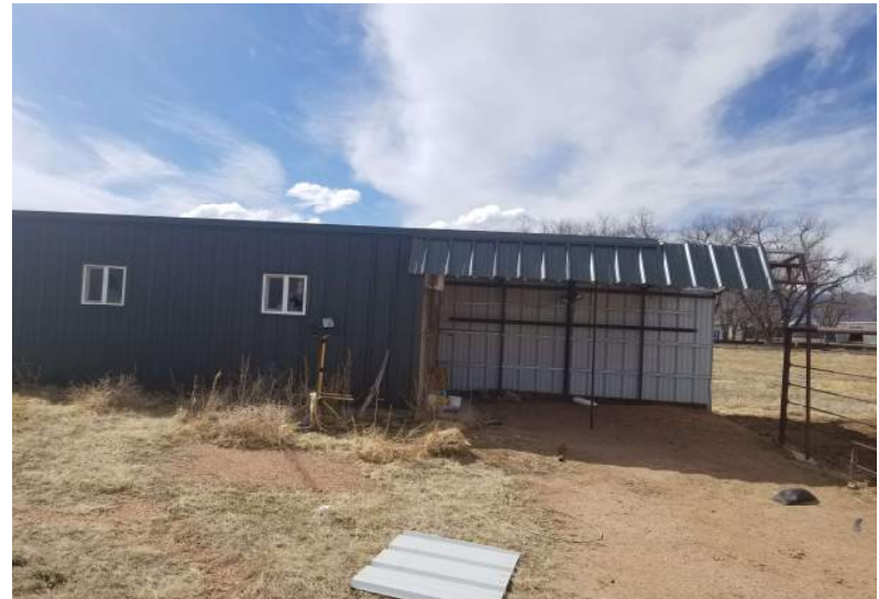
8. Structure on southwest corner of property.
