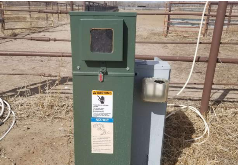
11. Electric box located near the southwest corner of Equestrian Center.
