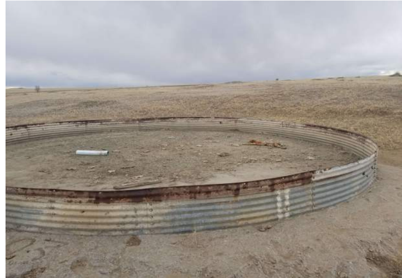
41 Stock tank southeast center of property.
