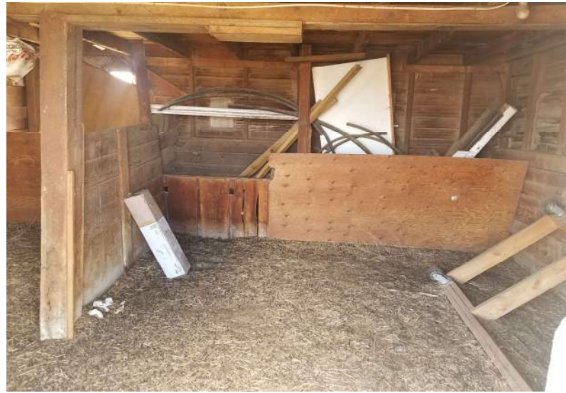
4. Interior of stable located near northwest corner of property.
