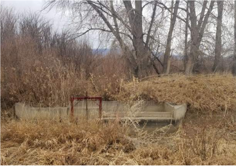
44 Sluice gate on southwest center of property.
