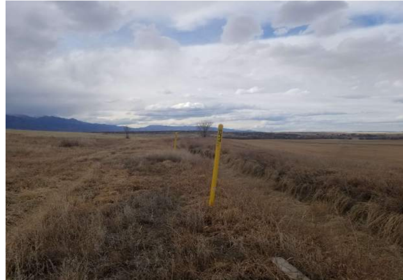
45 Gas pipelines along irrigation canal along the southwest center of property.
