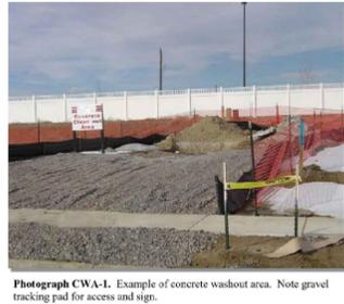
Photograph CWA-1. Example of concrete washout area. Note gravel tracking pad for access and sign.
