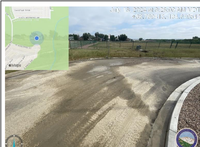
Photo 3: Remove sediment from driveway in front of building
