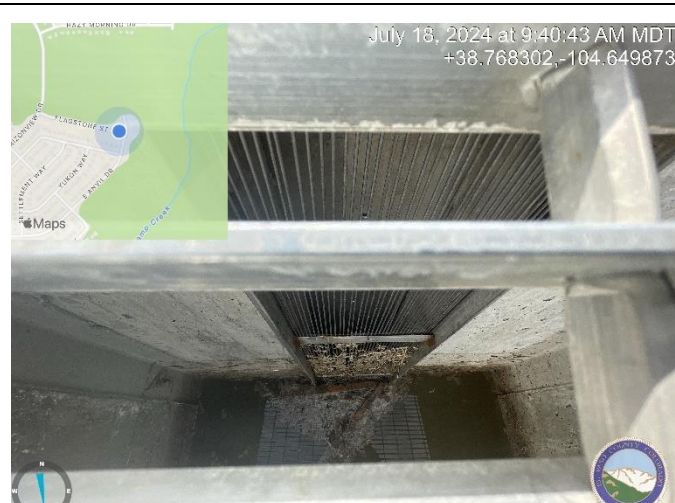
Photo 7: Microscreen not the correct material. Plans call for Johnson Vee Wire.
