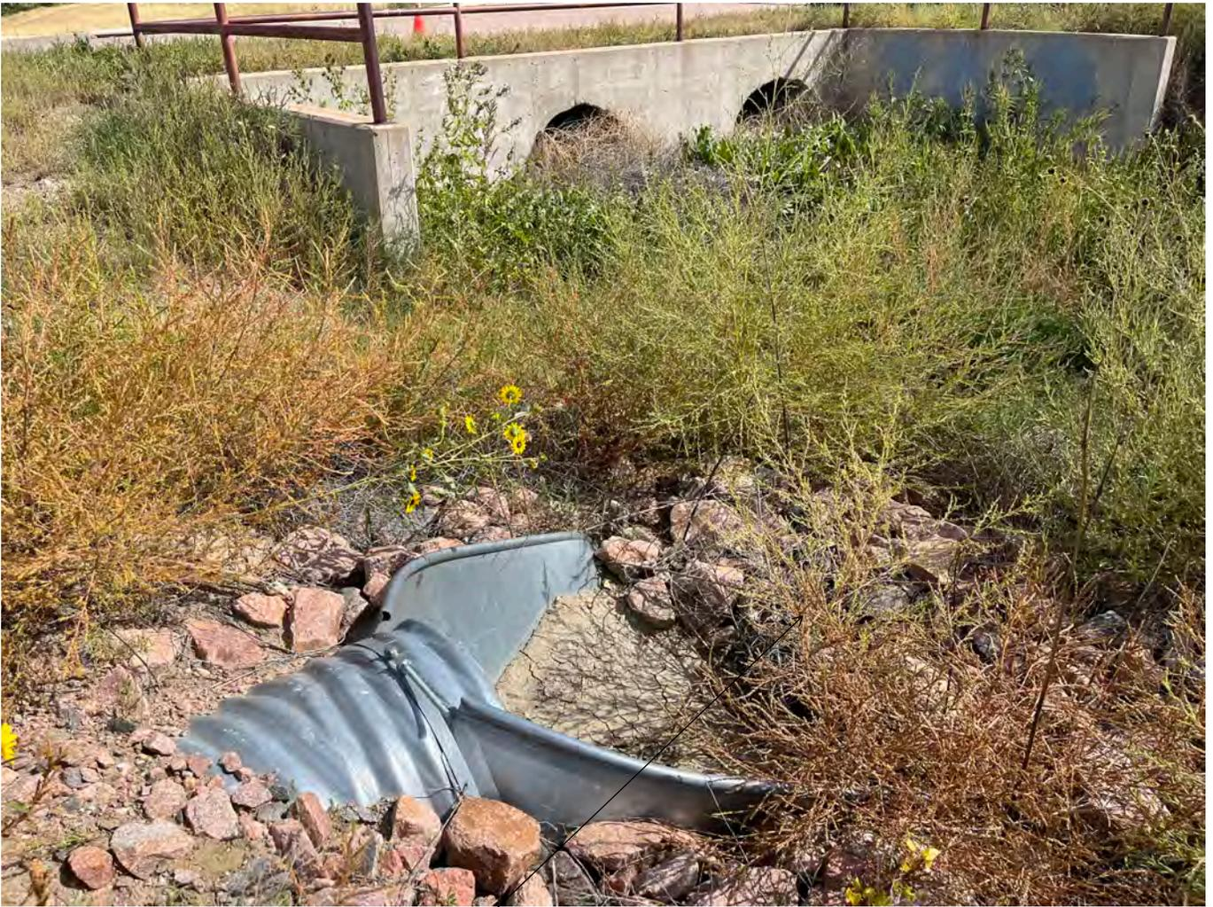
**Image taken looking southeast at the existing outfall configuration of the 24" CMP storm sewer line beginning onsite and terminating in Flagstone Channel.**
