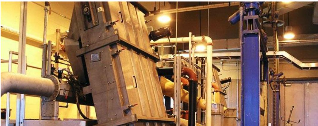
Typically bar screens fall under two classification, mechanical bar screens and manual bar screens (trash racks can either be manually cleaned or mechanically cleaned). Both manual and mechanical screens contain equally spaced vertical or inclined bars that span the width of a channel.
