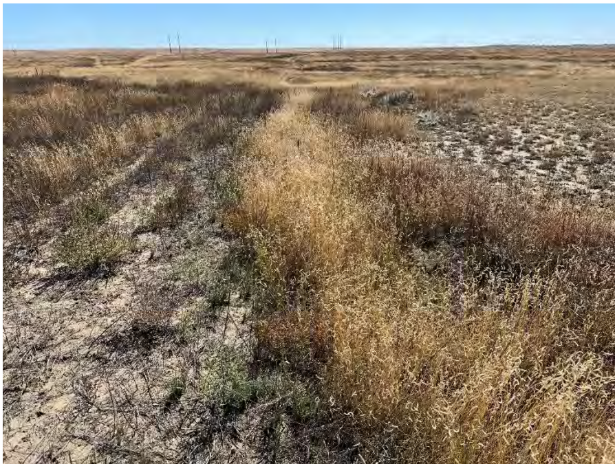
Photo 8: Representative photo of an earthen dam, dividing the channel.
