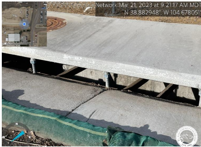
Photo 5: Remove forms and clean out sediment from curb inlet east of extended detention basin.
