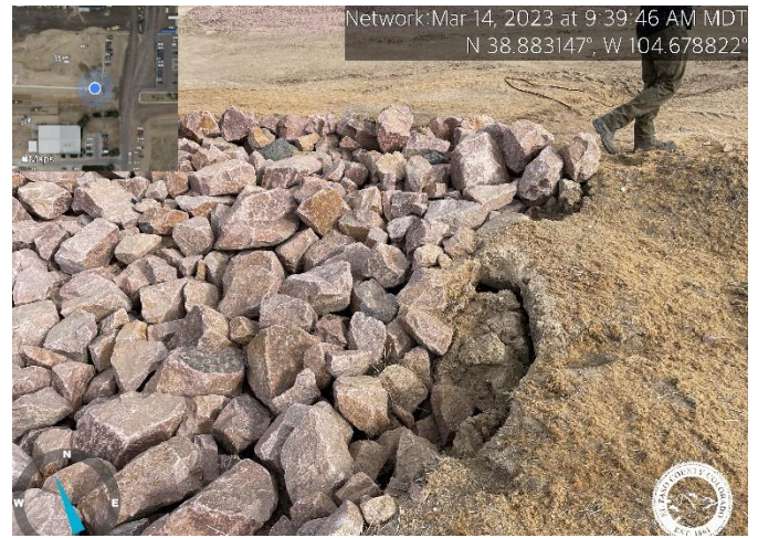
Photo 6: Address settling of riprap rundown at central forebay.
