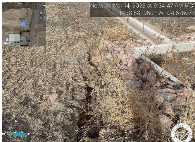
Photo 7: Repair rill erosion and implement final stabilization around eastern-most forebay.
