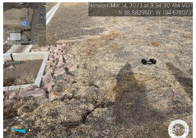
Photo 8: Repair rill erosion and implement final stabilization around eastern-most forebay.
