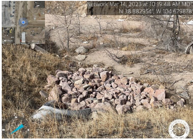
Photo 9: Low tailwater basin not installed per plan sheet ST03. Design engineer needs to provide revised design and calculations.
