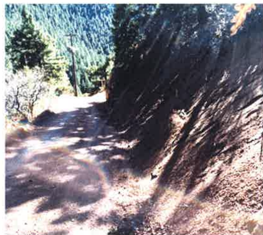
Camelot Road below building site
